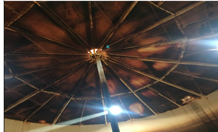
Greentree: Severe center column erosion
