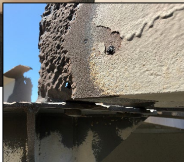
Metal loss/erosion
